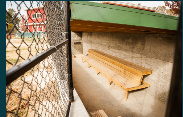
Improvements to local ball fields like the Watson Field underground dugouts in Clifton are just one of many things that can be funded by having permanent funding available.
